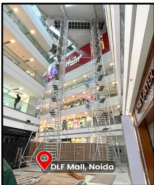
Rental supply of Aluminium Scaffolding (Model MS 134) at DLF Mall of India, Noida
